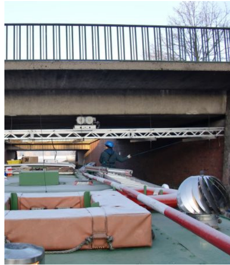
Figure 8: Examination of bridge girders.
