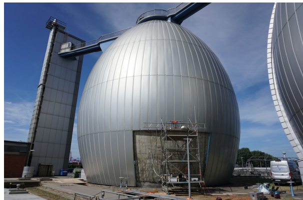
Figure 12: Examination of tendons of a digester.
