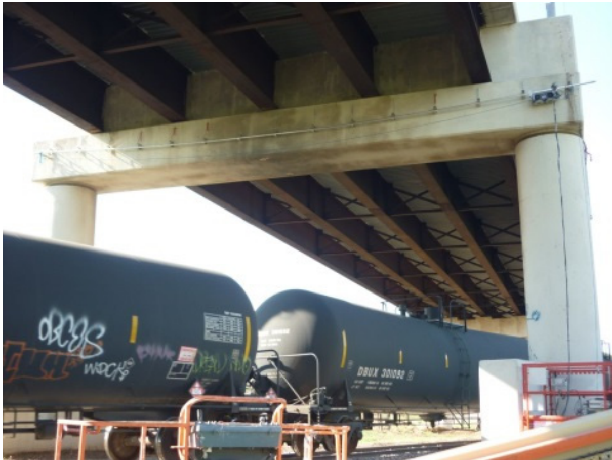
Figure 13: Examination of bridge girders with parabolic tendons.
