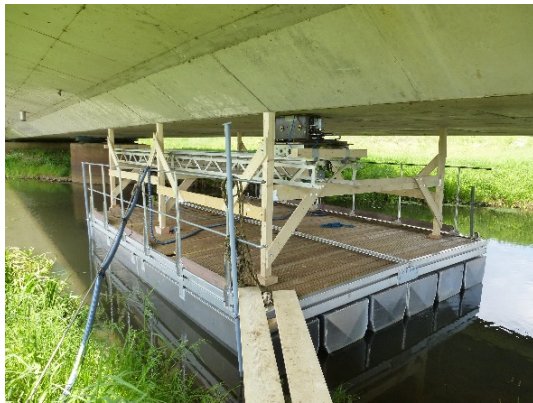
Figure 9: Examination of a prestressed concrete bridge with the help of a floating platform.
