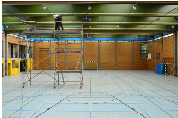
Figure 10: Examination of prestressed concrete girders in a sports hall.
